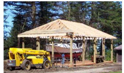
Building the framework for the housing.
