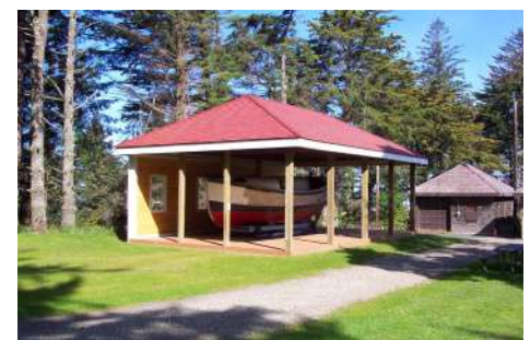
The final structure is complete. Note the bright red shingles. 2003.
