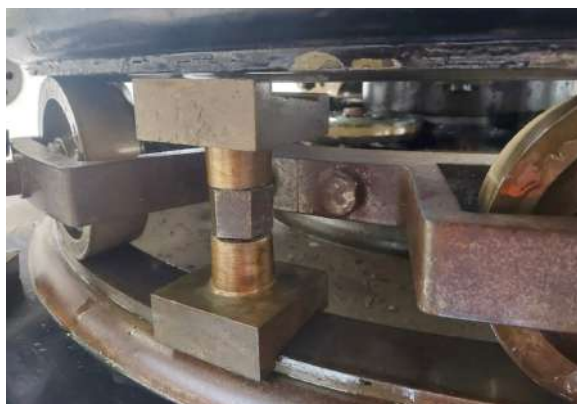
IN SEARCH OF: CBHS is currently searching for jacks similar to the ones shown in this photo for lifting the Fresnel lens to access the bearings.
